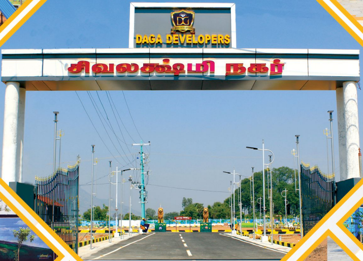
Entrance Arch with gated community
